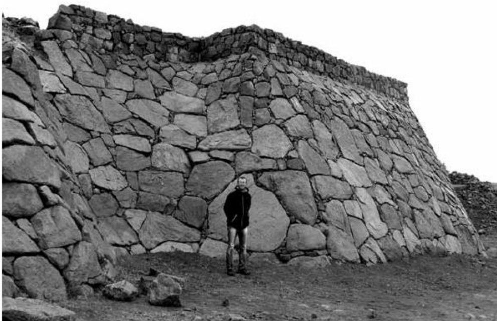
Figure 18. Restored section of the Cappadocia Gate glacis and wall
